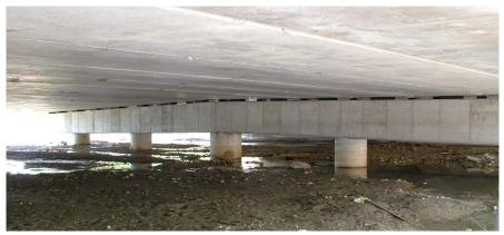
Box beams were selected to reduce the structural depth, and allow passage of the 100-year flood elevation with minimum impact to the existing approach roadway elevations.
