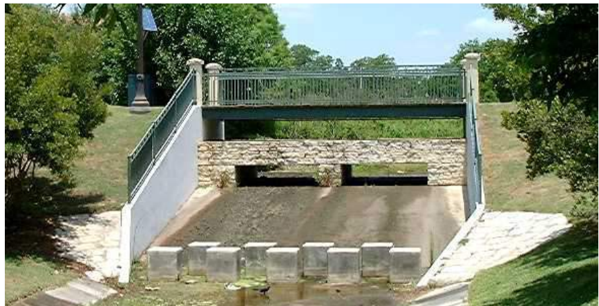
The lower pedestrian bridge is a single span structure spanning between the walls of a concrete outlet structure. Both bridges are 8 feet wide.
