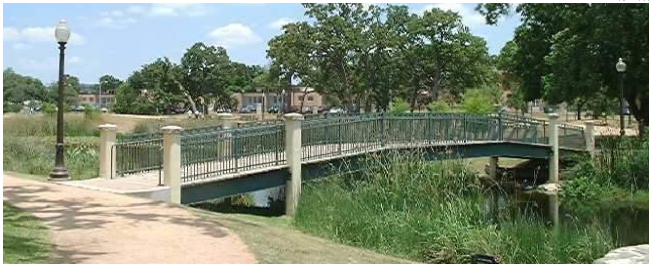
The upper pedestrian bridge is a 3-span structure with steel stringers and timber decking on concrete footings. The center span is segmented.
