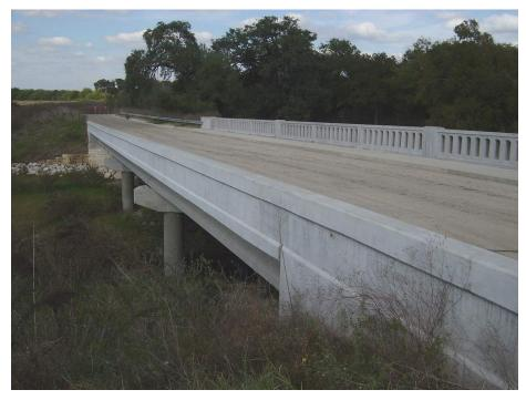
abutments and bents are skewed 68° to the roadway. AASHTO Type B prestressed concrete beams were used for all spans. A TxDOT T201 railing was selected as the traffic barrier, and a C411 railing was used adjacent to the sidewalk.
