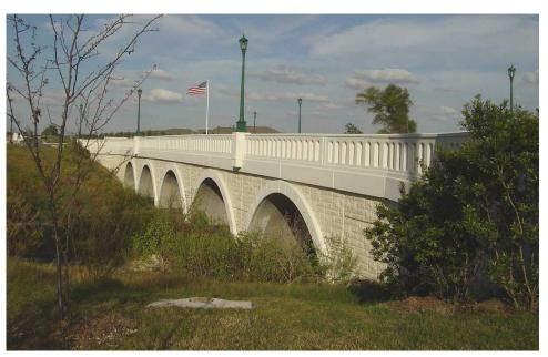
bridge length totals 148 feet. The bridge includes a 6-foot wide pedestrian sidewalk on both sides of the roadway, and has a total deck width of 50 feet.
