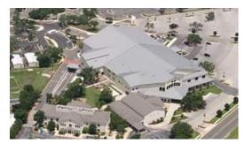
The building cladding consists of masonry at the lower floor, and a combination of metal siding and EIFS at the upper floors.
