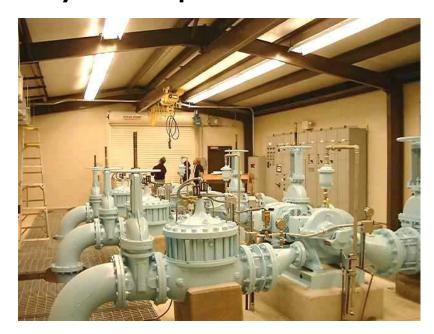
Pickett, Kelm & Associates, Inc. designed this 2,400 square foot, 5800 GPM pump building for LCRA in Dripping Springs, Texas. The building consists of a decorative masonry clad pre-engineered metal building with a prefinished metal roof. A ¾-ton electric hoist and trolley and removable grating panels over recessed pipe trenches were provided inside.
