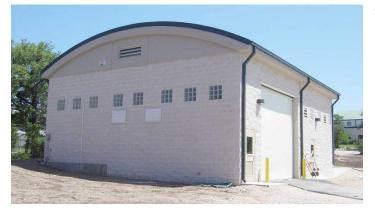
The structure consists of reinforced and fully-grouted load-bearing CMU walls. Steel bowstring bar joists support the barrel vault roof with a standing seam pre-finished metal skin. The foundation consists of a concrete slab-on-ground, with continuous perimeter grade beams and interior stiffening grade beams. Exterior cladding consists of a combination of split-face concrete masonry, EIFS and glass block.
