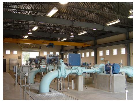
The superstructure consists of steel beams and columns supporting steel bar joists. Bowstring joists support a barrel vault roof over the pump room. CMU shear walls and moment resistant steel frames provide lateral bracing. The foundation consists of a concrete slabon-ground, thickened at each pump, with drilled piers founded in limestone at the column locations.
