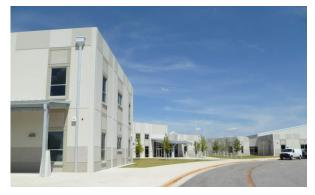
classroom floors, and second floor framing consists of composite slabs supported by composite steel framing. Lateral resistance to wind loads at the classroom pods is provided by braced steel frames.
