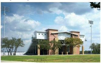
The pressbox encloses approximately 3,450 square feet and consists of a steel framed gabled roof and a composite concrete and steel framed floor supported by steel columns and two towers consisting of concrete tilt-up wall panels, topped by hipped roofs, and exposed galvanized steel trusses. The tower panels are clad with thin brick.
