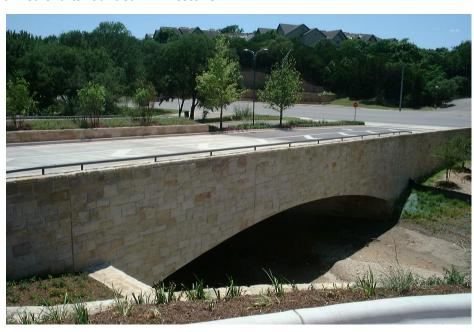
Standard concrete bridge railings were faced with stone veneer and topped with a decorative steel pedestrian rail. An arched stone veneer façade, supported by secondary steel framing, conceals the bridae superstructure. Curved mechanically stabilized earth wingwalls, with decorative stone facing, were provided at each corner of the bridge.
