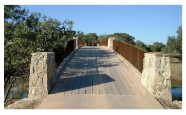
and two 45-foot approach spans are supported by variable depth arched weathering steel trusses. The substructure consists of reinforced concrete bents and abutments supported by concrete piers. The bridge received a Merit Award in the 2003 National Bridge Competition from the National Bridge Alliance and AISC.
