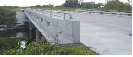
foot minimum width sidewalk on one side of the roadway and a 10.5 foot minimum width hike and bike path on the other side, for a total deck width of 70 feet.
