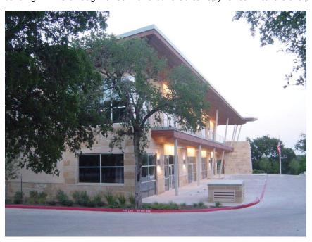
The building superstructure is steel-framed with open-web bar joists at the roof and a concrete slab over composite steel beams and giders at the floors. Exposed sloping steel tube columns support the structured second level walkway and cantilevered Lateral resistance to wind roof. loads is provided by moment frames. The foundation consists of perimeter concrete basement walls on grade beams founded in limestone. Straight-sided drilled shafts support interior column loads.
